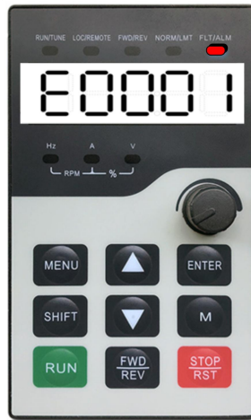
Figure 6-1 Interface fault display
